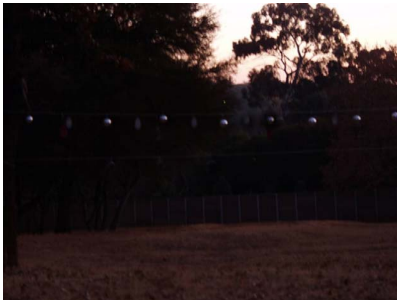
Figure 5: A Reflective Bird Diverter (left) installed on a line with conventional bird flappers (right).
